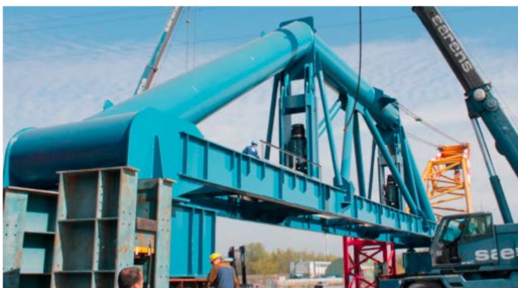
LIFTING BEAM O.V. SARENS NV
