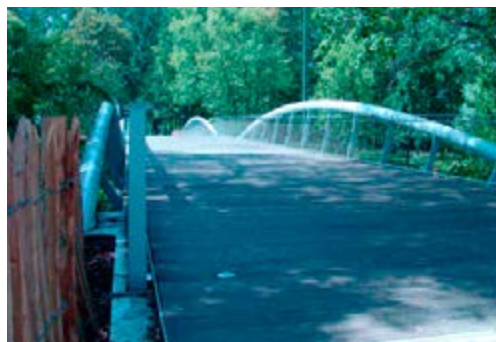
PASSERELLE / ANDERLECHT: NOMINATION 2012
